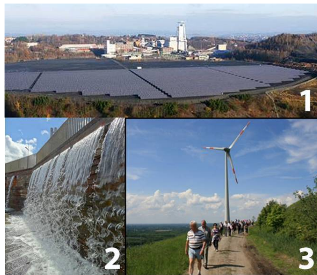
Figure 8 – Creating Renewable Energy, an Opportunity of Post-Mining. 1 Photovoltaic plant on a mud pond; 2 Heat from mine water; 3 Windmill on a dump
